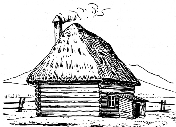
Figure 4: Russian bathing establishment from the governor Yaroslav. Similar to the Finnish sauna houses, the Banja is also built from logs in block construction. As an advance over the "smokehouse", this bath already has a fireplace.
